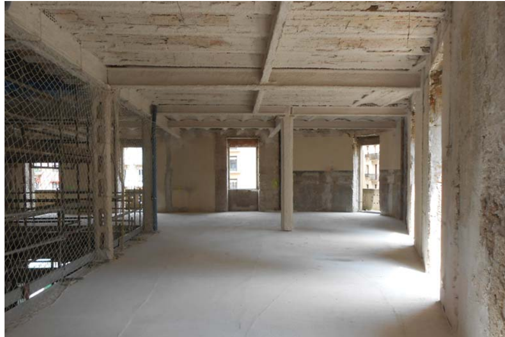
Metal structure on the second floor.
