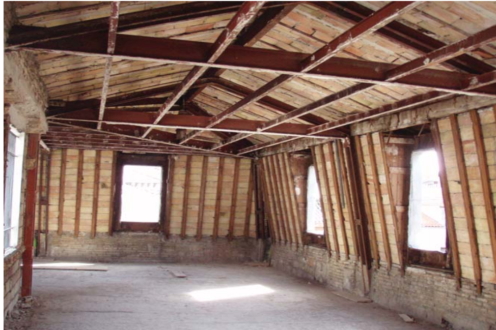
Old roof structure.
