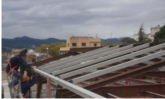
Roof metal structure.
