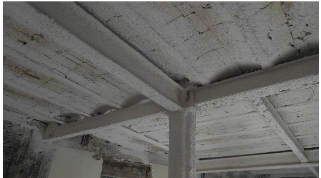
Fireproof protection on metal structure.
