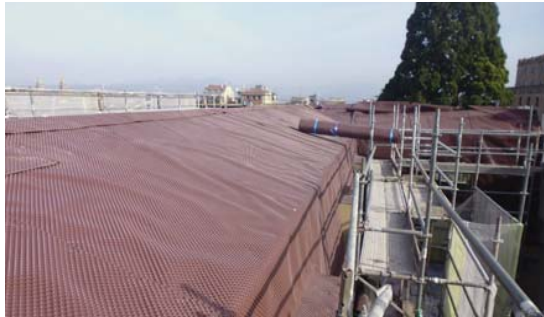
Roof covering system.
